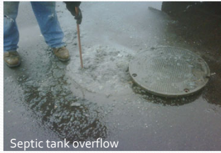
Septic tank overflow
